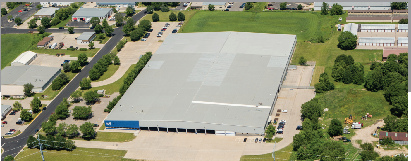
Middleton, WI ■ 220,000 Square Feet ■ 2115 Pinehurst Drive
