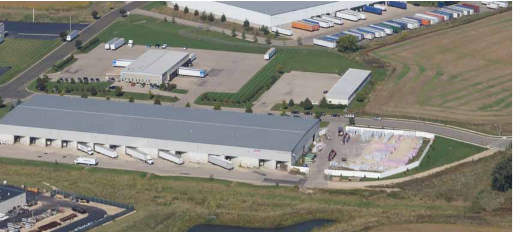
101,800 SQ. FT. HIGH-BAY DISTRIBUTION CENTER IN DEFOREST, WIS.
