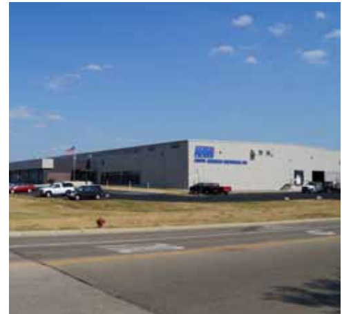
LEED-CERTIFIED OFFICE AND MANUFACTURING BUILDING ALONG HIGHWAY 19 IN BURKE, WIS.
